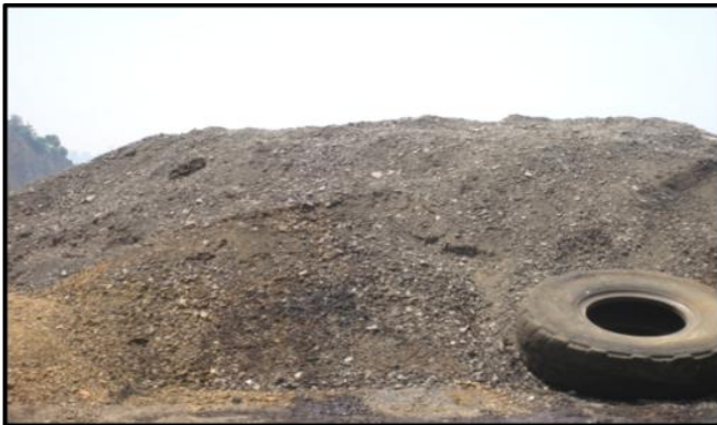
Fig. 2. Milled Asphalt Dumped for Backfilling at Dbayeh Marina.
